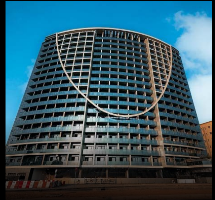
The V Tower Dubai Land
