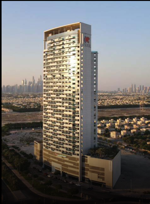
Al Jawahara Tower JVT, Dubai
